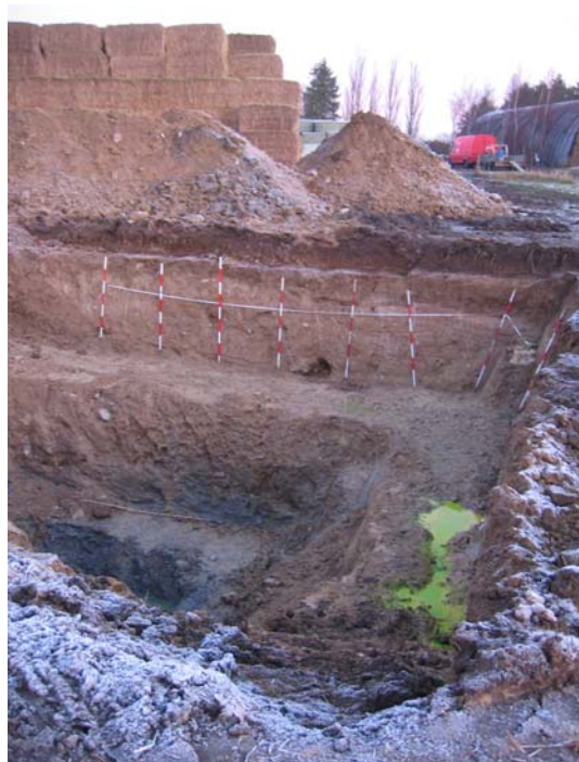
Figure 5.4: Photo of the excavation carried out at the Vasby site, December 2005. Looking North. The NE corner of the site described in Københavns Amt (2005a; 2005b) is located by the red truck and barn seen in the photo.
